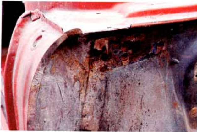
Trapped debris and moisture were certainly the culprits for the rust that affected this area where the front subassembly bolts to the cowl.
