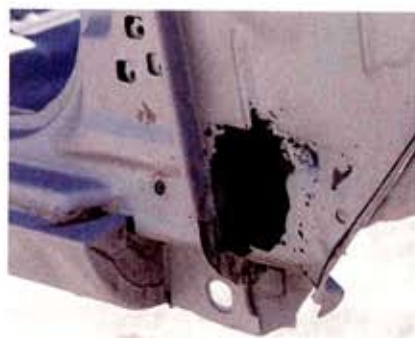
The bottom of the cowl on both sides was rusted through in this rust-prone area. Blasting made a very minimal change in the size of the hole, demonstrating the gentle impact that the IB Mineral has on the metal. Careful inspection will reveal how much metal has to be cut out and replaced.
