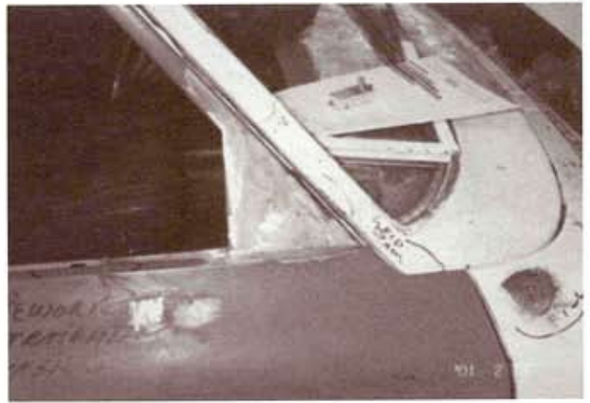
Eliminated vent glass and built panel and window channell for base for custom made mirrors.
