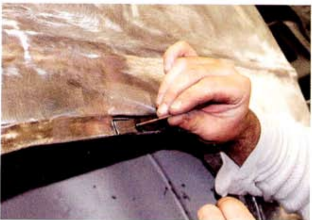
15 A small patch of metal is hard to handle, so Rock used a stud gun to attach a stud to the metal. By doing so, it can be held properly during welding.
