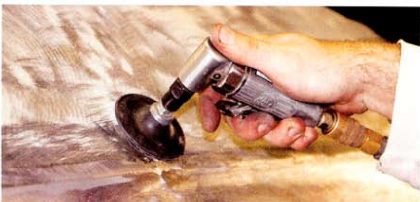
19 When the metal was where it needed to be, the stud was cut off and ground smooth. This method is far superior to drilling holes into panels in order to accomplish the same result.
