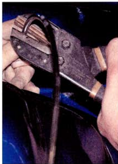
The airlines are cut to length allowing for a clean installation.
