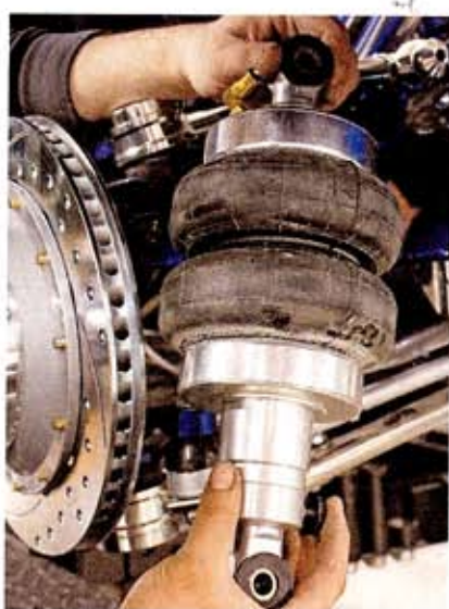
The ShockWaves are slipped into position for installation.
